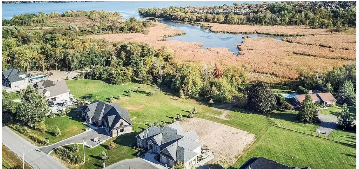
Figure 15: Castle Harbour Drive, looking southeast
