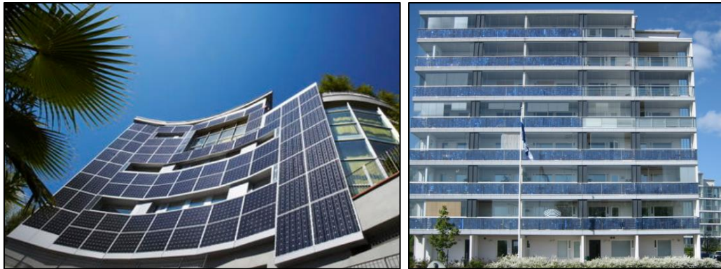
Figure 6: Building Integrated PV System
