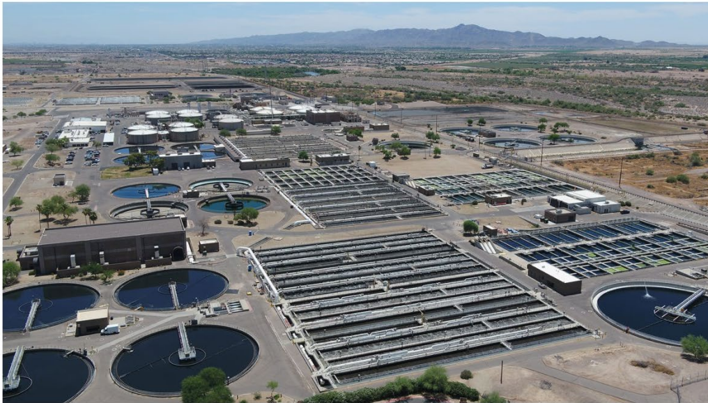
An aerial view of Phoenix's 91st Avenue Wastewater Treatment Plant. Phoenix Water Services Department
