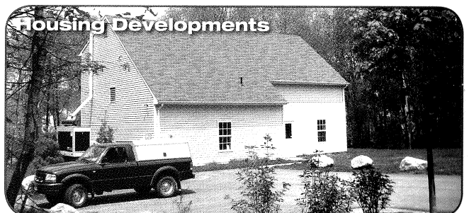
Country Oaks, NJ – 50,000 GPD. Decentralized wastewater treatment plant serving a 166-unit residential development.
