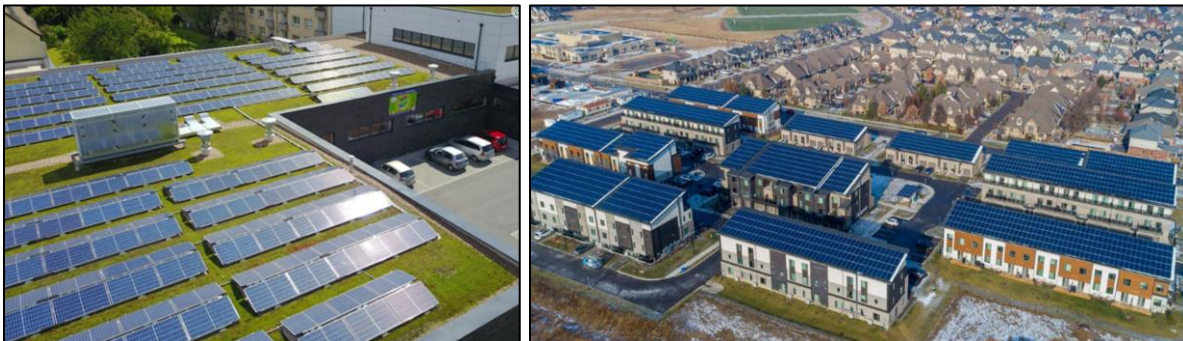
Figure 5: Rooftop Solar PV System
